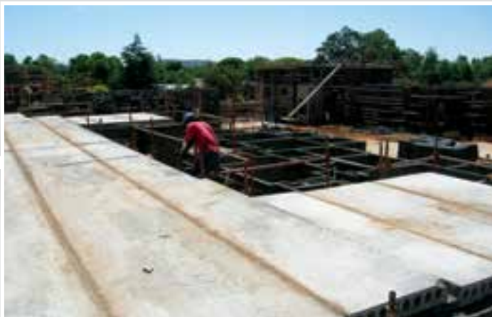
The grouted slab, building can continue once the grouting has cured.
