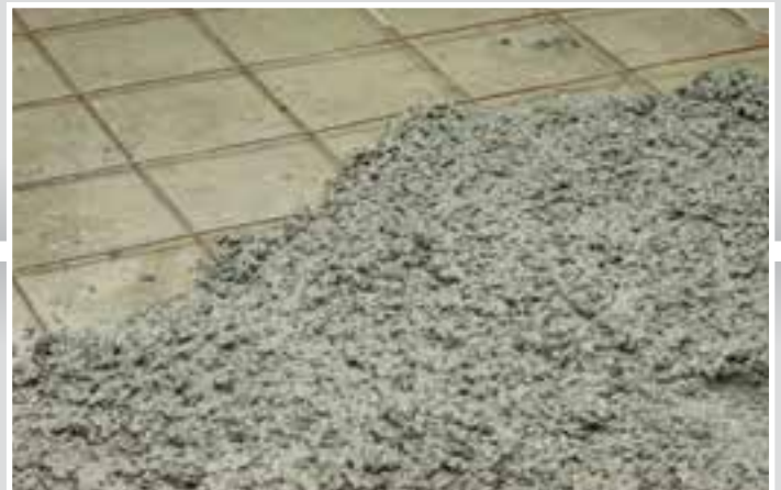
Mesh in screed / topping by the contractor.
